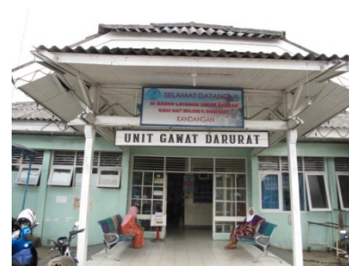
Kandangan Hospital (Indonesia)
